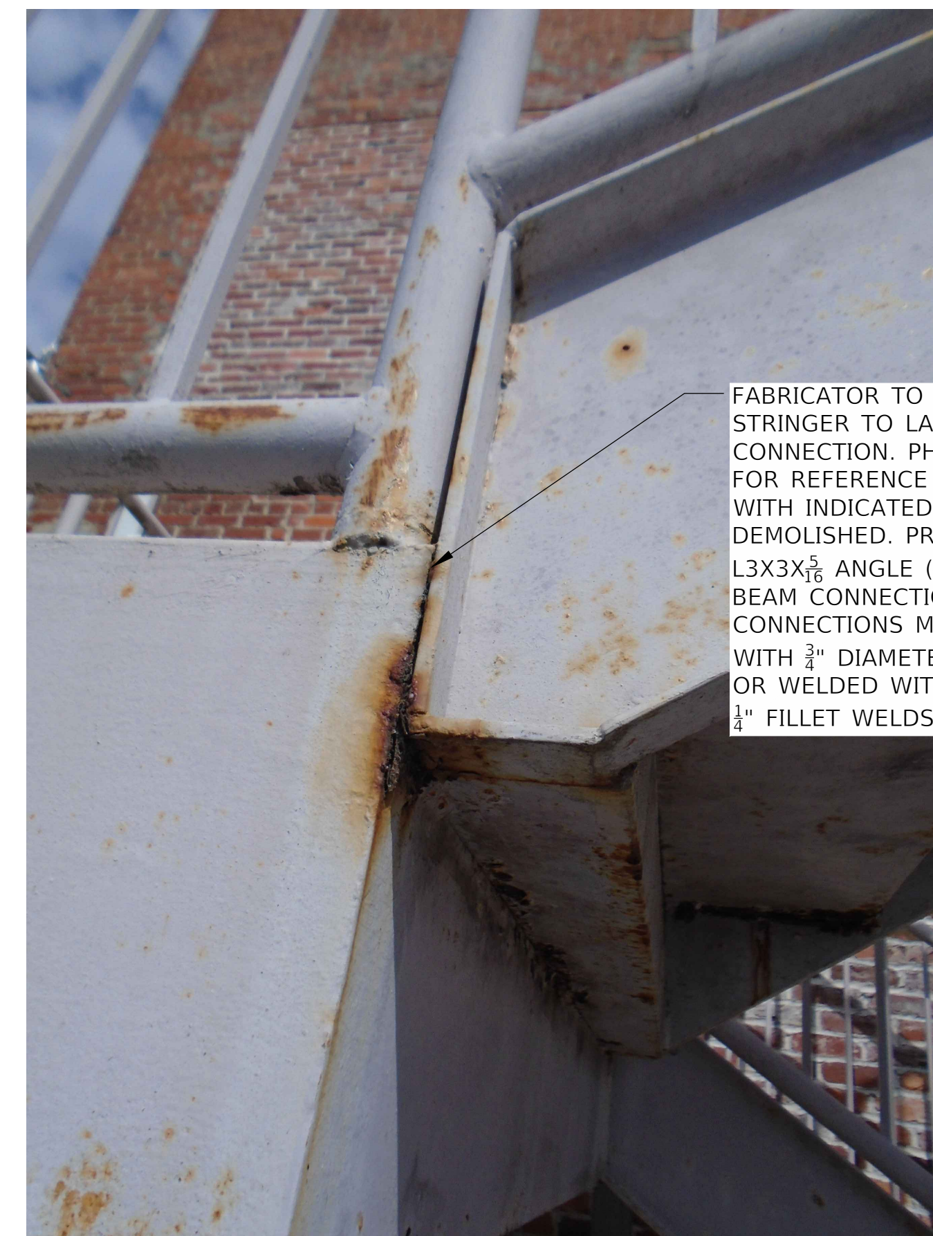
F STRINGER CONNECTION TO LOWER LANDING REPAIR PHOTO DETAIL
