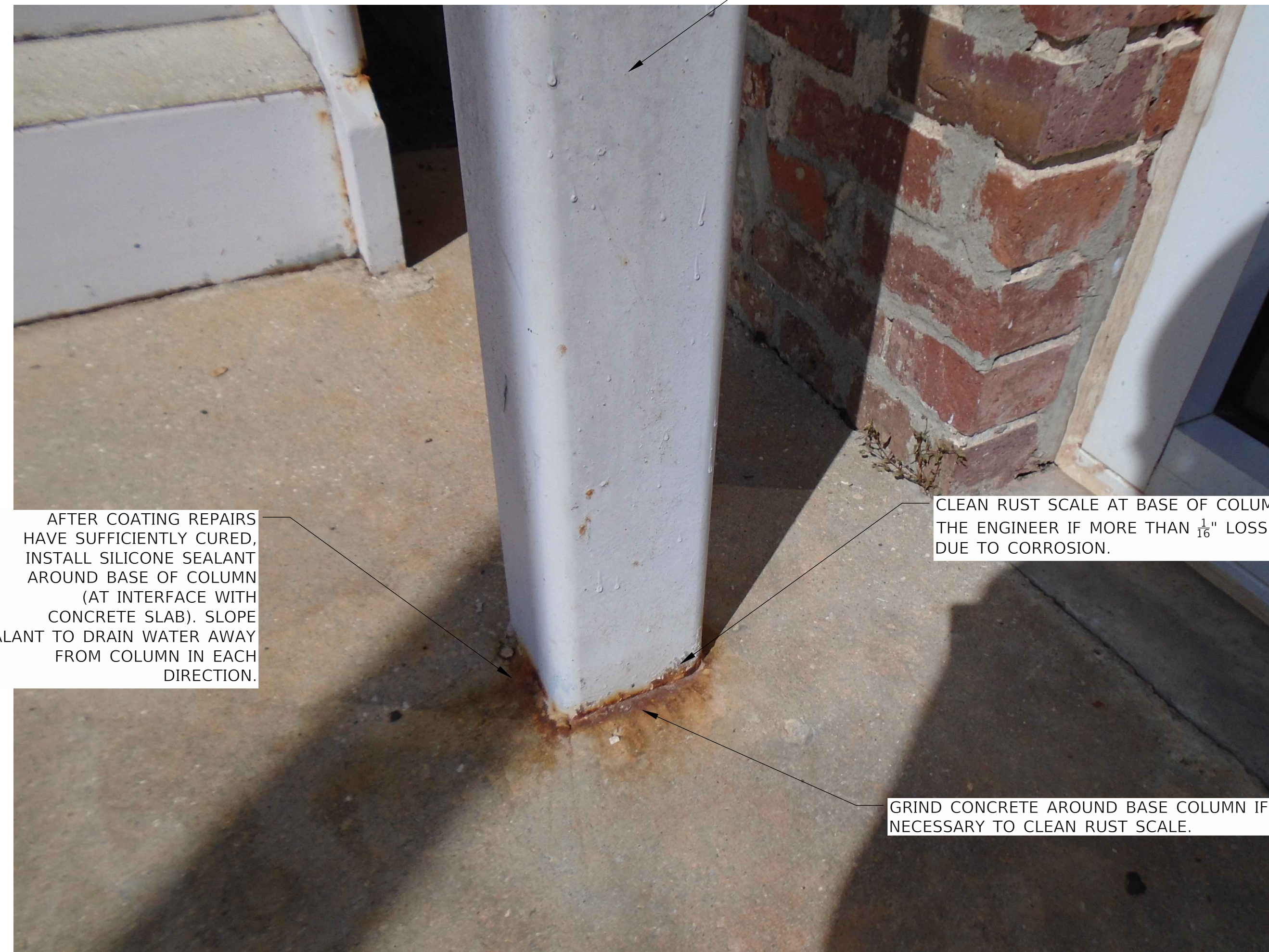
A TYPICAL CORRODED COLUMN BASE REPAIR PHOTO DETAIL SCALE: N.T.S.
