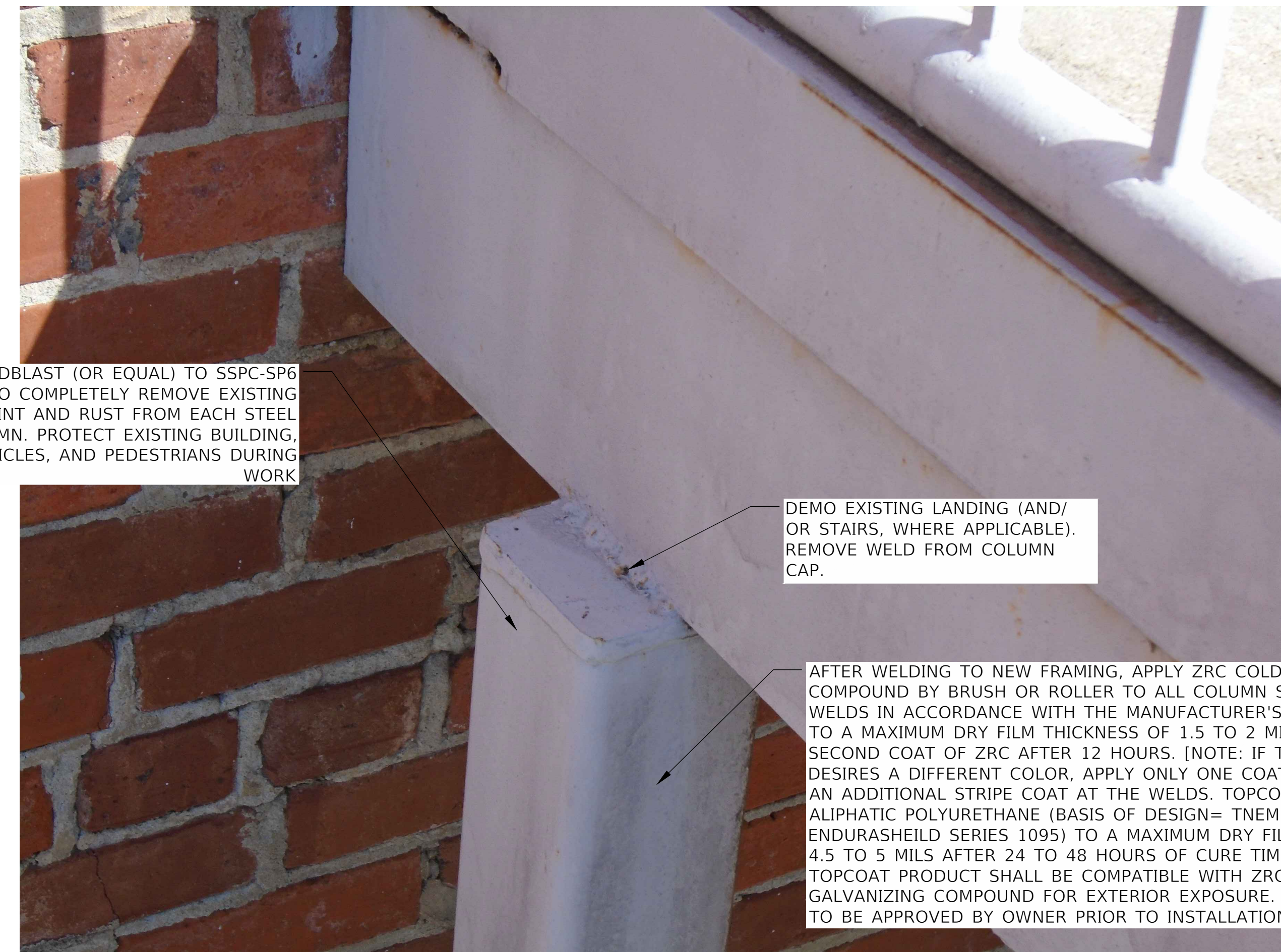
B TYPICAL COLUMN CAP REPAIR PHOTO DETAIL SCALE: N.T.S.
