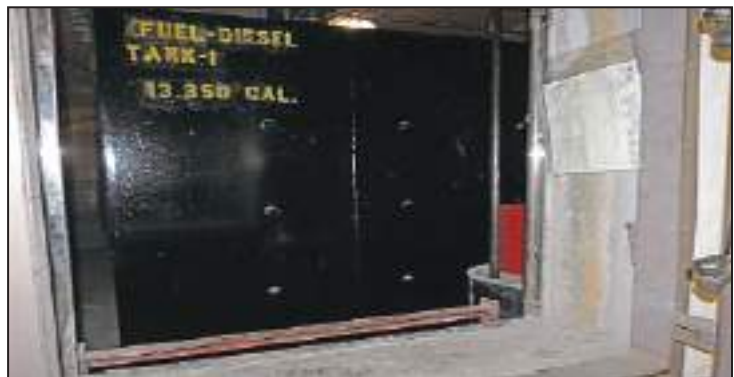
Figure 5-23. Fuel tank placed in floodproof vault in basement of commercial high-rise (New York, NY).
