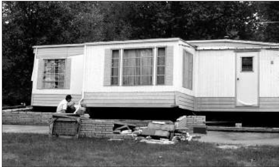
Figure 5-6. Failure due to sliding.
