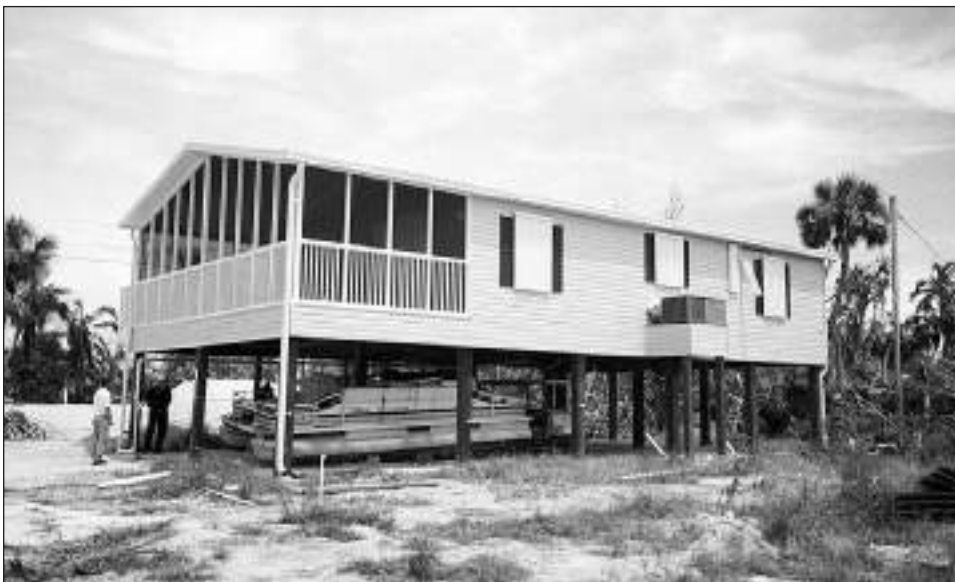
Figure 8-4. Manufactured home on a pile foundation.
